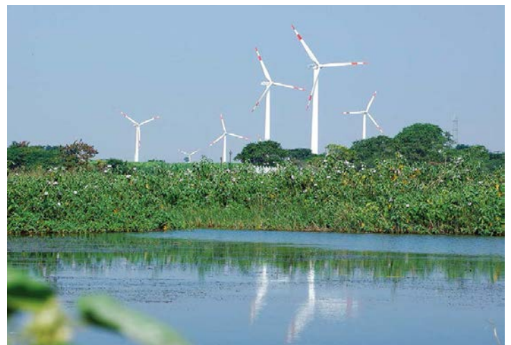
Fig. 12. Wind farm in Dhule, Maharashtra
